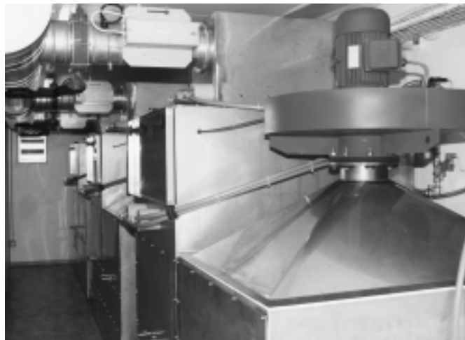
PLASMACAT units with integrated fan
